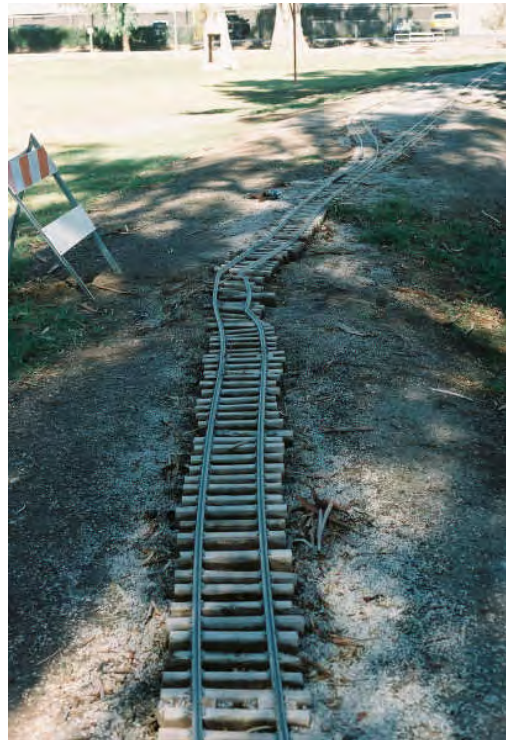
Track damage at Joe Henry Park in July
