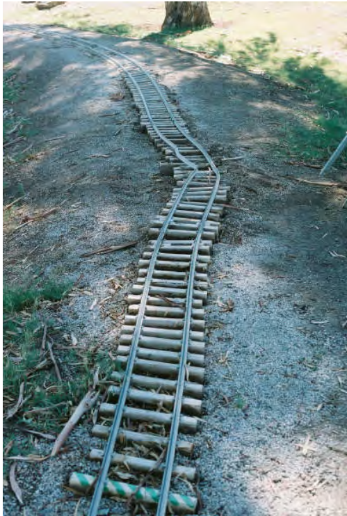
Track damage at Joe Henry Park in July
